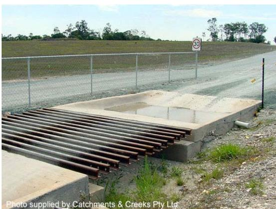
**Photo 5 – Vibration grids are usually located prior to a wash bay**
