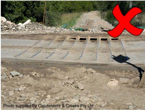
**Photo 7 – Heavy sediment build-up on a construction exit**
