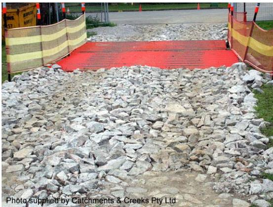
Photo 1 – Vibration grid and rock pad
