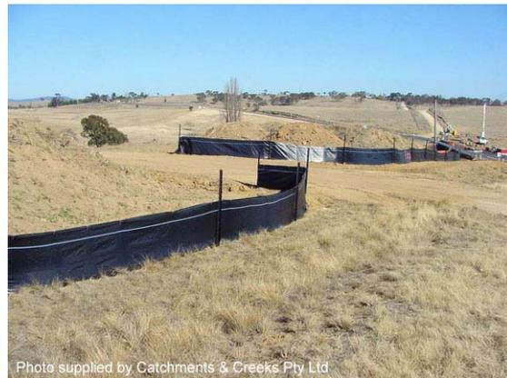
Photo 2 – Sediment fence placed down-slope of soil stockpile
