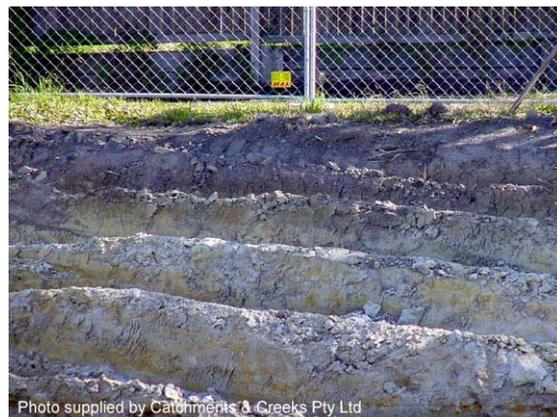
**Photo 4 – Stair stepping of step batter**
