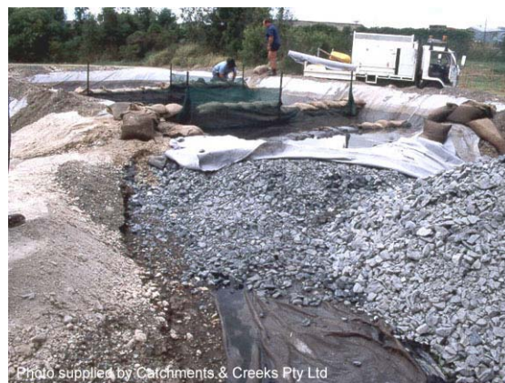
Photo 3 – Rock-lined overflow spillway
