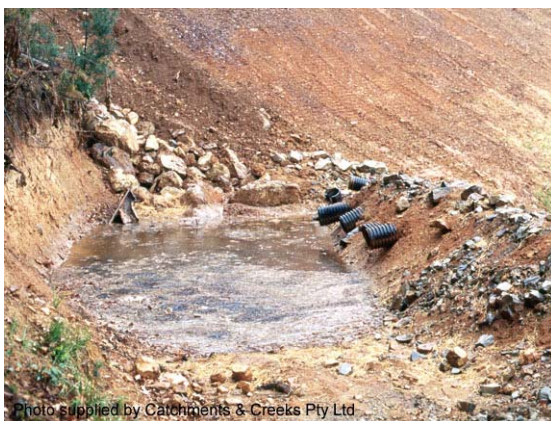
Photo 2 – Siphon pipe overflow system
