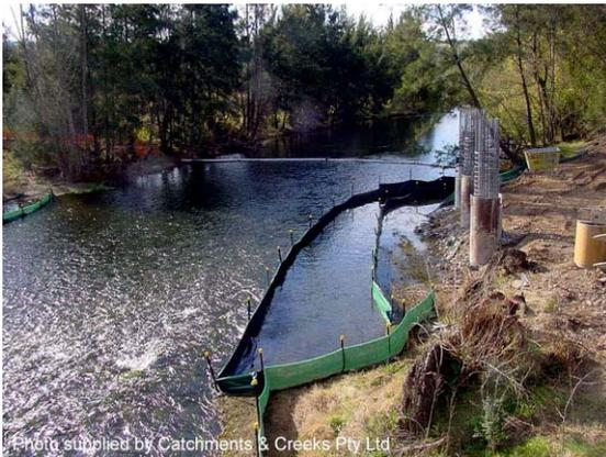
Photo 1 – Sediment fence isolation barrier with landward sediment fence
