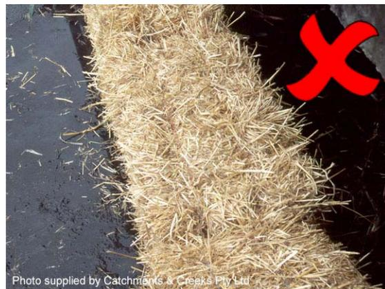
**Photo 2 – Straw bales should not be installed without a filter cloth wrap unless their operational life is less than 1 day**
