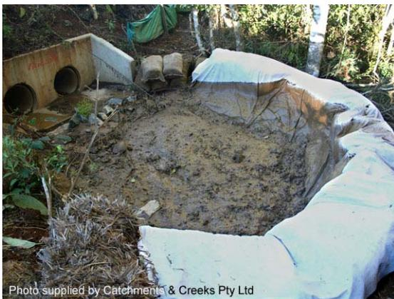
**Photo 1 – A supplementary straw bale barrier placed up-slope Type-2 sediment trap (not in picture)**
