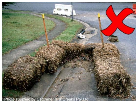
**Photo 6 – Straw bales should not be staked into road surfaces**
