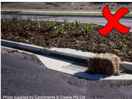
**Photo 5 – Straw bales should not be placed on solid surfaces**
