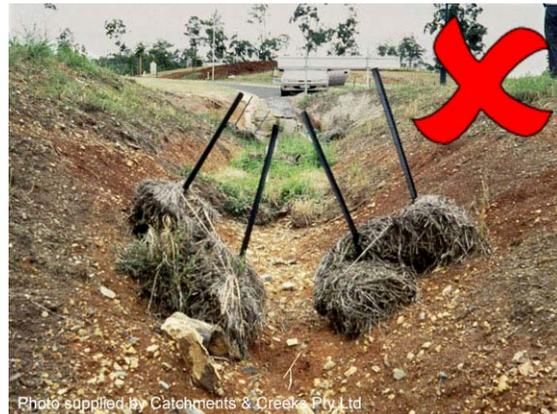
**Photo 4 – Once wet, straw bales readily fall apart resulting in failure of the structure**
