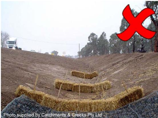
**Photo 3 – Straw bales should not be used to form check dam sediment traps**
