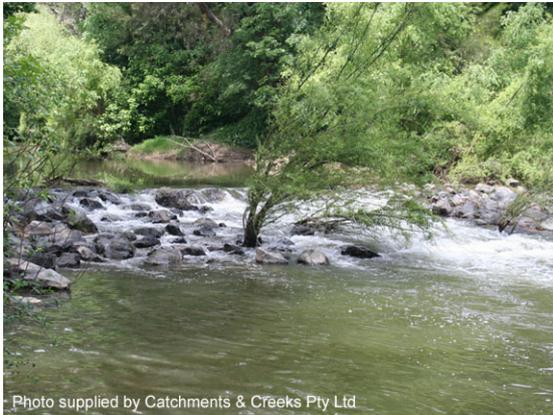
**Photo 1 – Constructed riffle**
