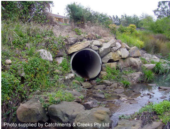
Photo 1 – Rock stabilised pipe outlet
