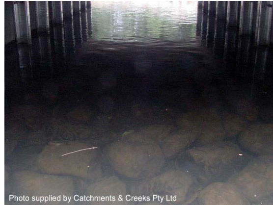
Photo 2 – Enhanced bed roughness along the base of a box culvert
