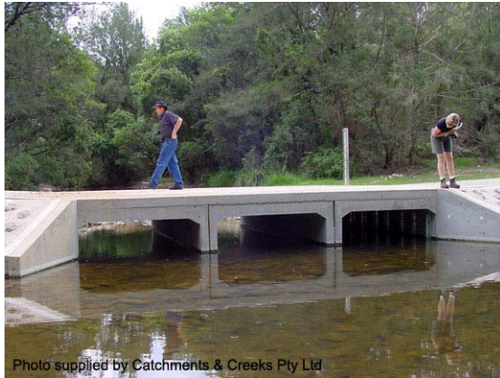
Photo 1 – Fish-friendly box culvert with roughened bed conditions
