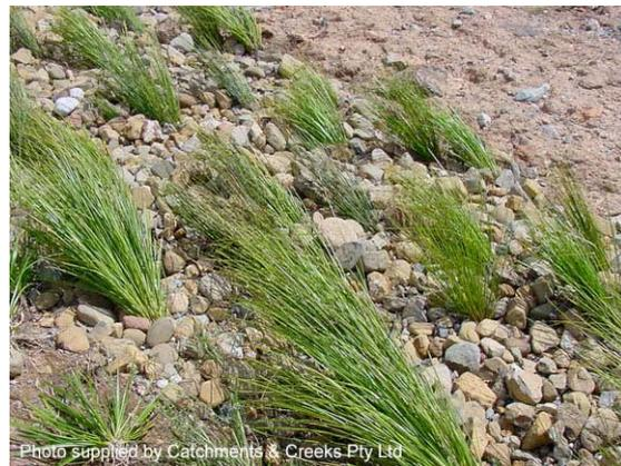
**Photo 2 – Rock mulching incorporated into stormwater bio-retention swale (post storm condition)**
