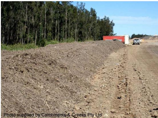
Photo 1 – Large mulch filter berm
