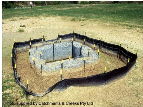
**Photo 2 – A *Sediment Weir* can be used as an alternative to a traditional mesh and aggregate system**
