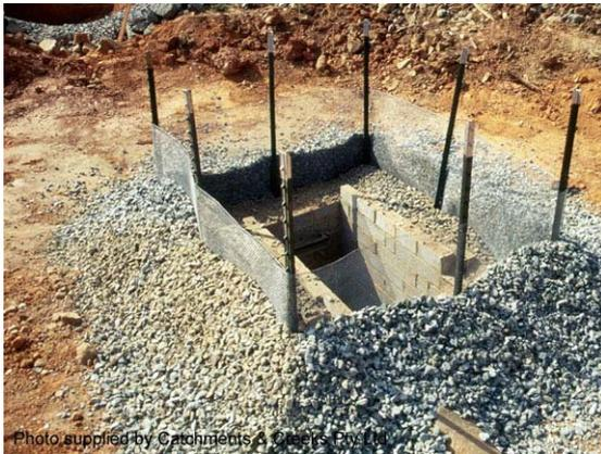
**Photo 1 – Mesh and aggregate drop inlet protection**
