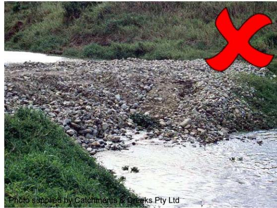
**Photo 4 – If operated for extended periods the rock embankment can become saturated with fine sediments resulting in sediment release into downstream waters**
