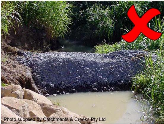
**Photo 3 – The rock embankment should not be made entirely from fine aggregate**
