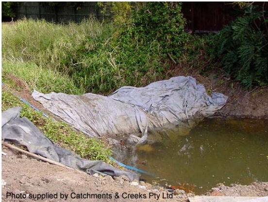
**Photo 1 – Rock filter dam with geotextile filter**
