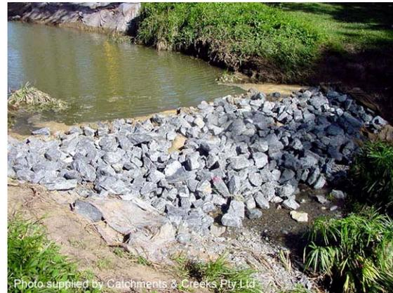
**Photo 2 – Rock filter dam with aggregate filter**
