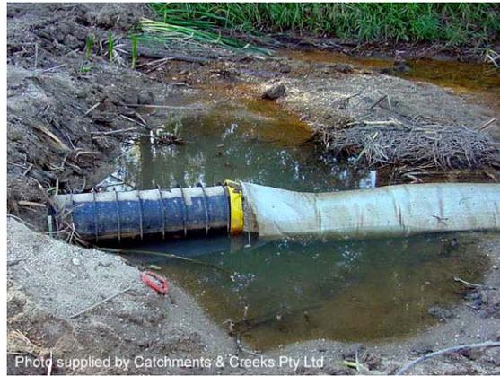
Photo 4 – Ribbed pipe used to anchor pipe within the earth embankment
