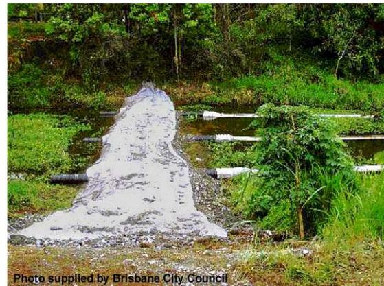
Photo 2 – Filter tube barrier
