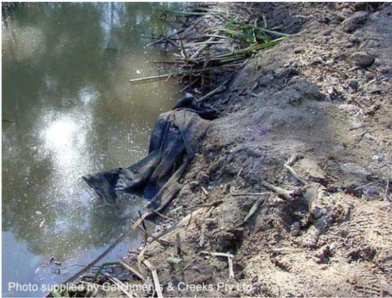
Photo 3 – Open weave fabric (e.g. shade cloth or wire mesh) placed over the pipe inlet to exclude aquatic wildlife
