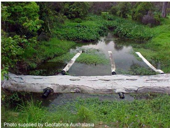
Photo 1 – Filter tube barrier
