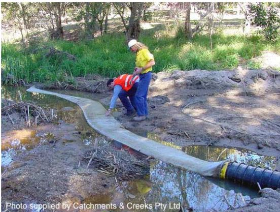
Photo 5 – Filter tube looking downstream
