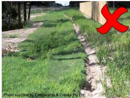
**Photo 4 – Undesirable rilling along edge of turf caused by lateral inflows**
