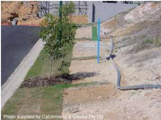
**Photo 5 – Lateral turf strips can reduce the risk of flow diversion along up-slope edge of turf**
