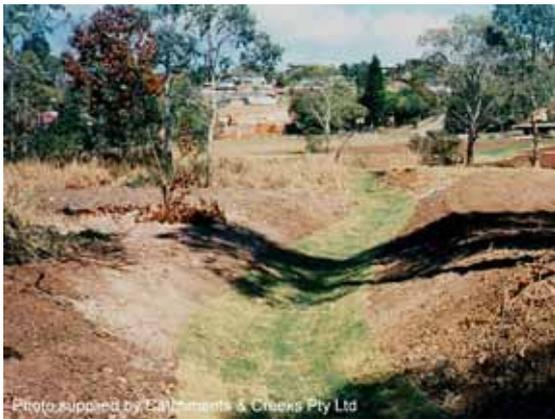
Photo 1 – Grass-lined flow diversion channel
