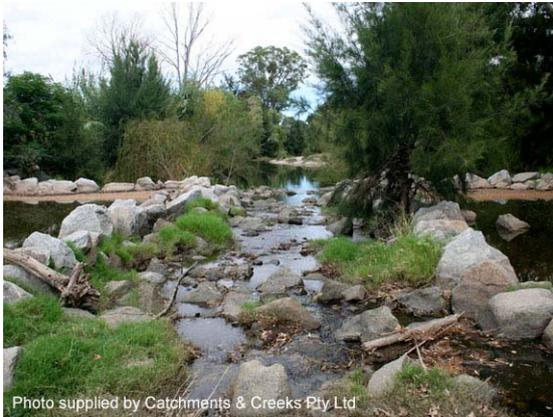
**Photo 1 – Rock chute/ramp fishway near Tamworth, NSW**
