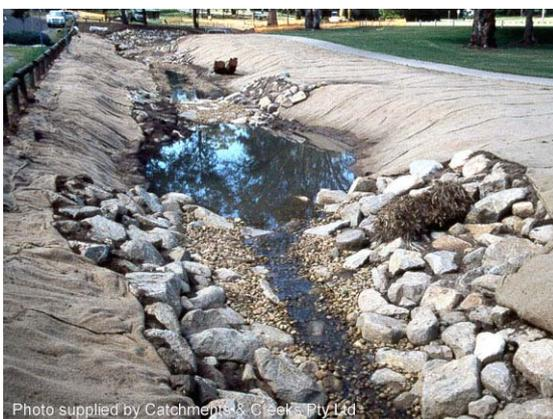
**Photo 5 – Constructed pool-riffle system**
