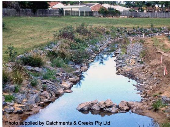
**Photo 4 – Early stages of revegetation of a rock stabilised stream bank**
