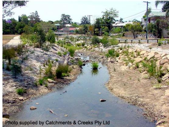
**Photo 2 – Rehabilitation of an old concrete stormwater drain, Brisbane, QLD**
