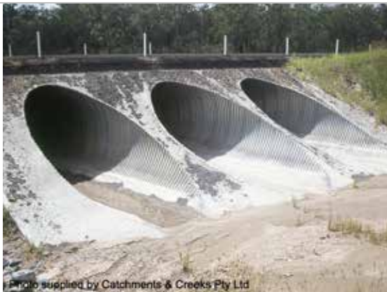
Corrugated steel pipe culvert
