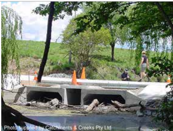
Post-flood culvert inspection
