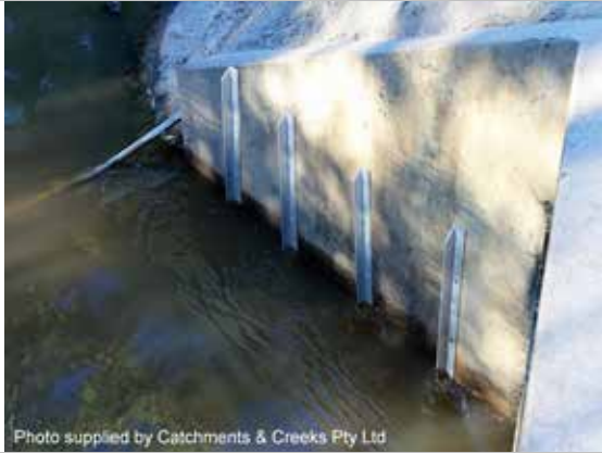
Baffles on upstream wing wall
