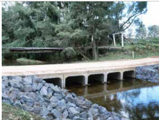
Box culvert with adjacent rock chutes
