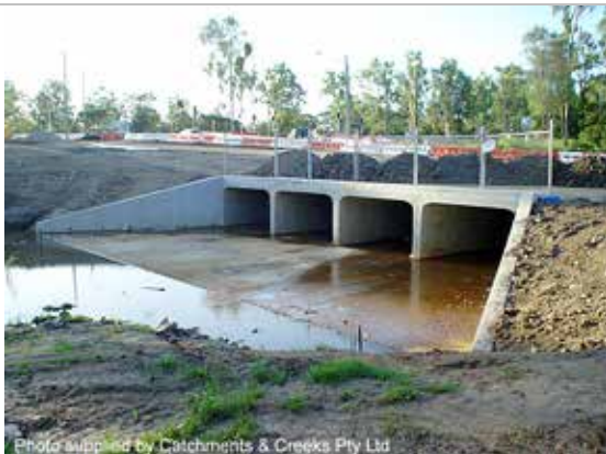
Lengthening of an existing culvert
