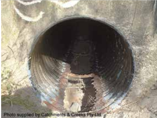
Culvert in need of maintenance
