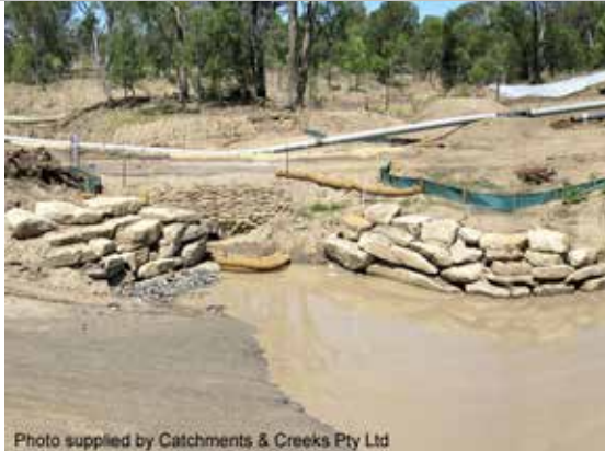
Photo supplied by Catchments & Creeks Pty Ltd
