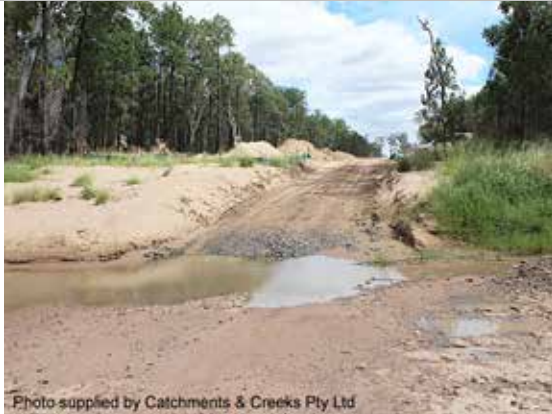
Ford crossing under construction
