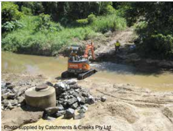
Maintenance to sewer pipe
