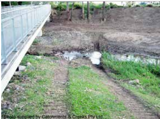
Temporary creek crossing
