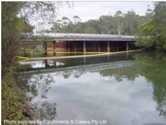
Temporary sheet piling in tidal waters
