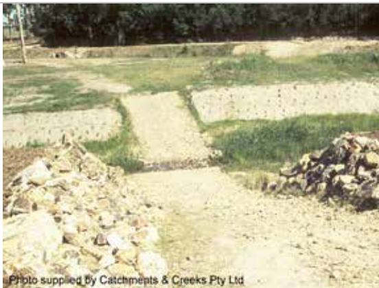
Site rehabilitation works
