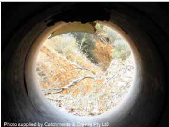
Failed concrete pipe lining
