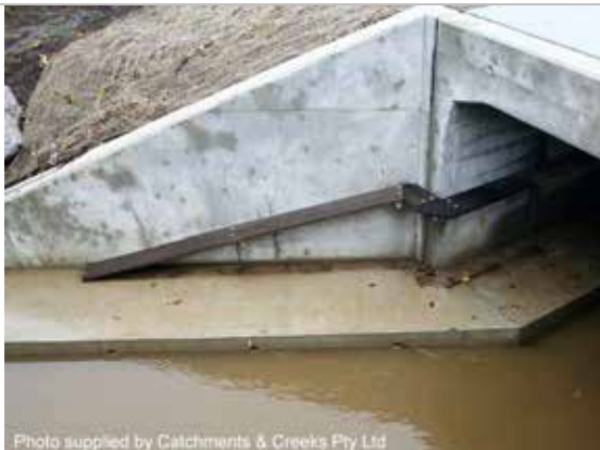
Box culvert with terrestrial pathways
