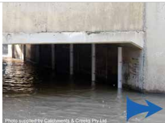
Sidewall baffles (looking upstream)
