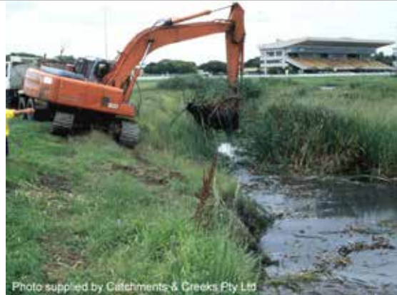
Drainage channel maintenance
