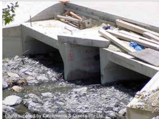
Headwall construction
