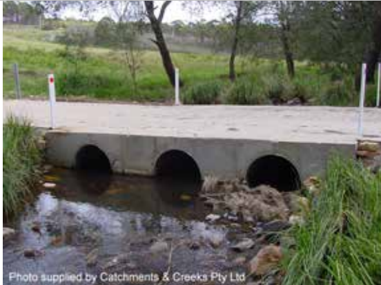
Recessed pipe culvert
