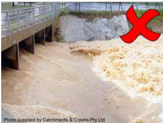
Excessive outlet turbulence
