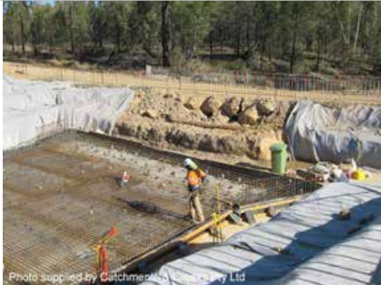
Photo supplied by Catchments & Creeks Pty Ltd Temporary road bypass
