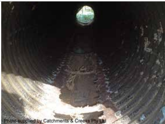
Culvert in need of maintenance
