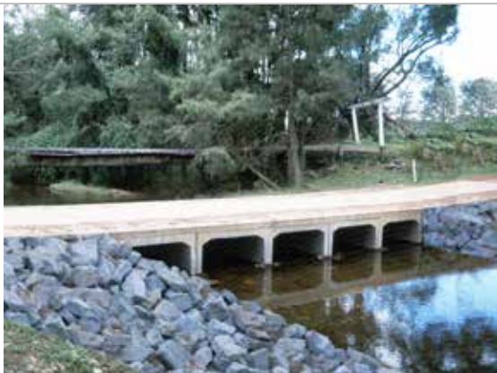
Option 3 culvert with rock chutes
