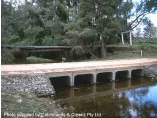
Recessed, low-level, rural culvert
