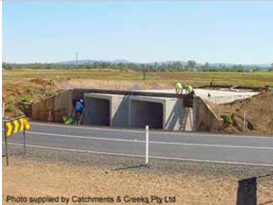
Culvert construction
