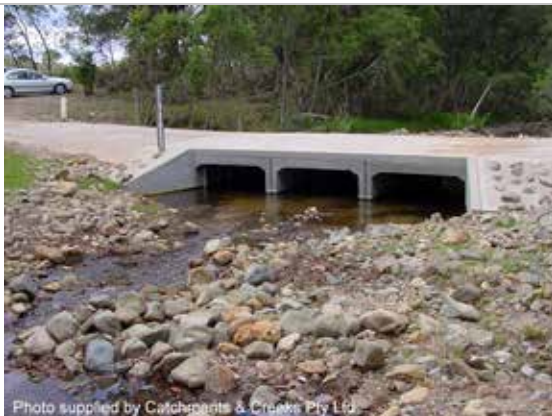
Recessed box culvert
