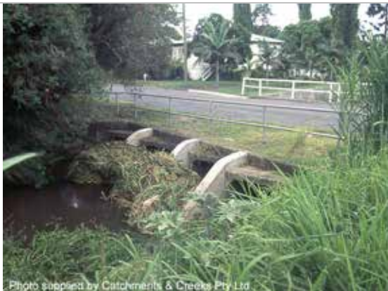
Debris caught on debris deflector walls
