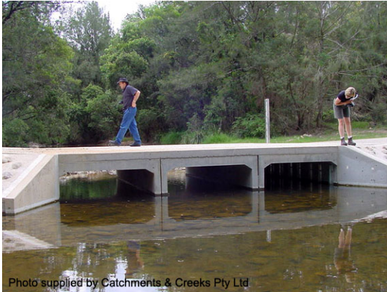
Backwater passing through a culvert
