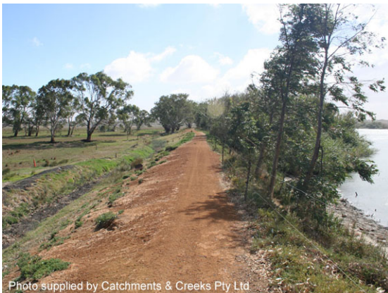
Flood control embankment (levee)
