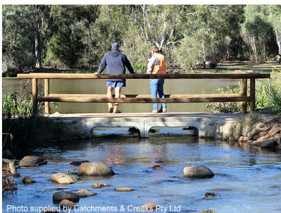
Outflow from swamp into bypass channel
