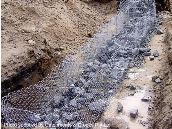
Gabion wall under construction
