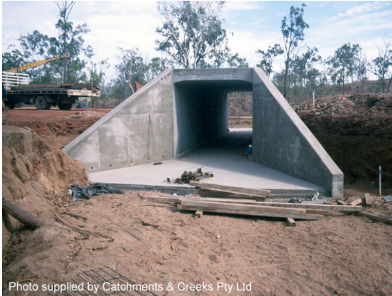
Culvert with wing walls under construction
