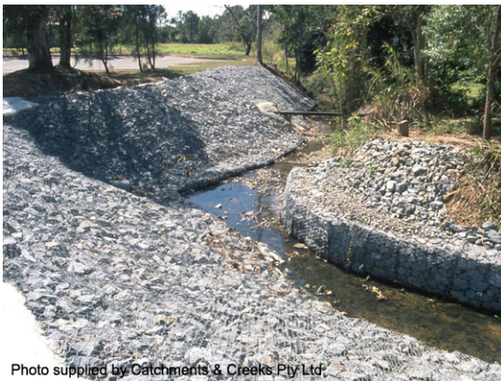
Channel lined in rock mattresses
