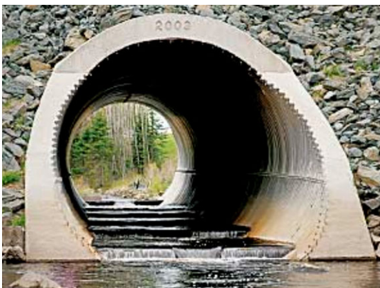
Notched shallow weir baffles
