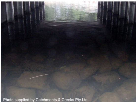
Rocky 'invert' of a fish-friendly culvert
