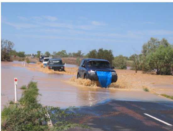
Limited trafficability of crossing
