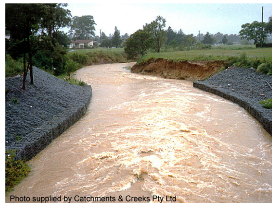
Wholly rough culvert outlet jet
