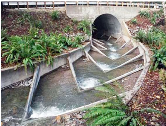
Chevron baffles at culvert inlet
