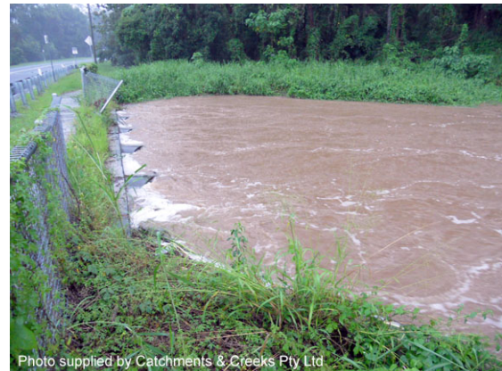
Culvert operation under outlet control
