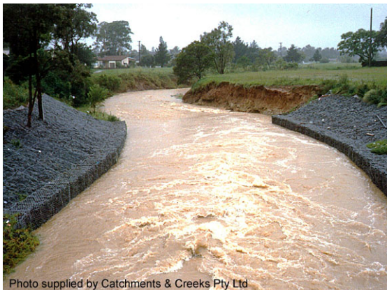
Outlet jetting from culvert
