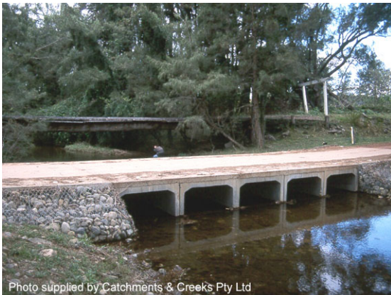
Culvert operation under outlet control
