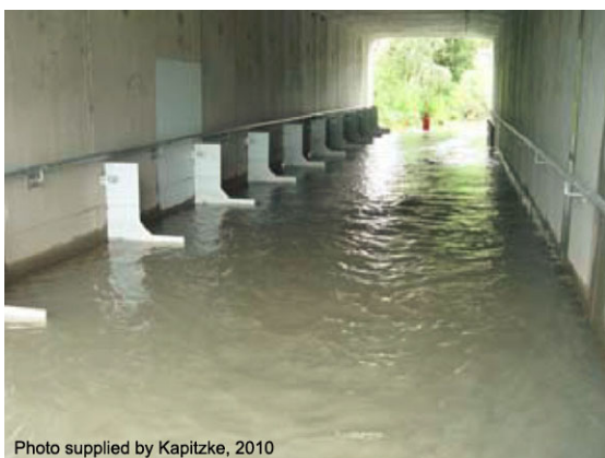
L-shaped corner baffles
