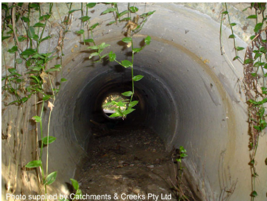
Pipe culvert barrel
