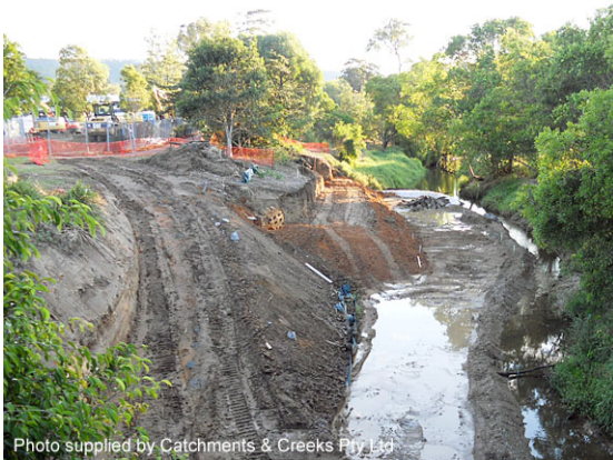
Placing fill adjacent to a creek
