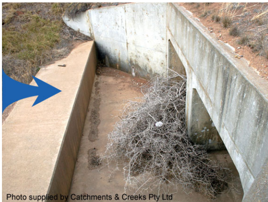
Culvert with a drop inlet
