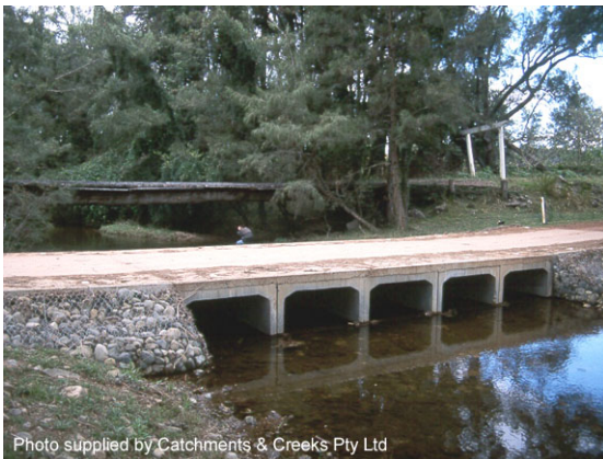
Recessed box culvert
