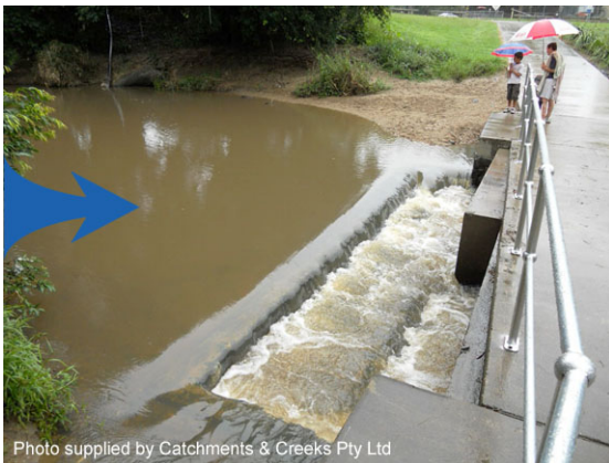
Operational culvert fishway
