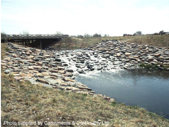
Grouted boulder drop structure
