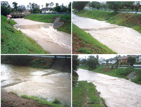
Four degrees of weir drowning
