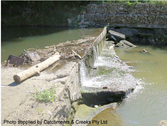
Fish passage barrier (weir)
