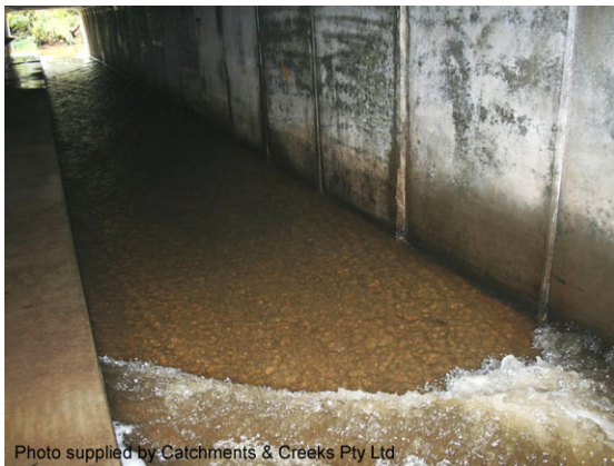
Supercritical flow (upstream of HJ)
