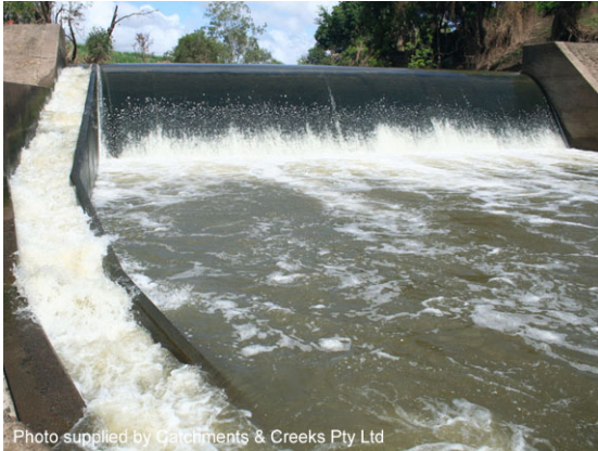
Fish ladder adjacent a weir
