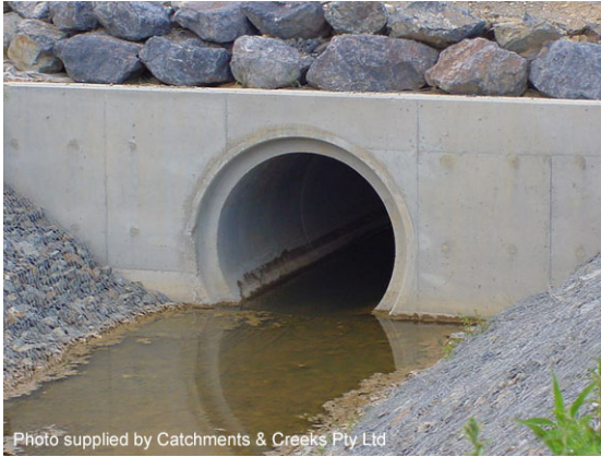
Single cell pipe culvert
