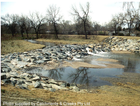
Grade control structure
