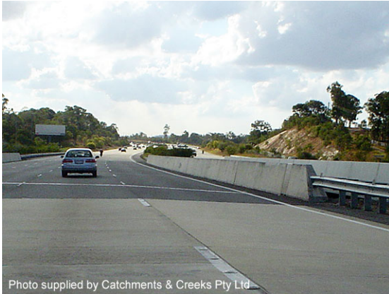
Major road bridge
