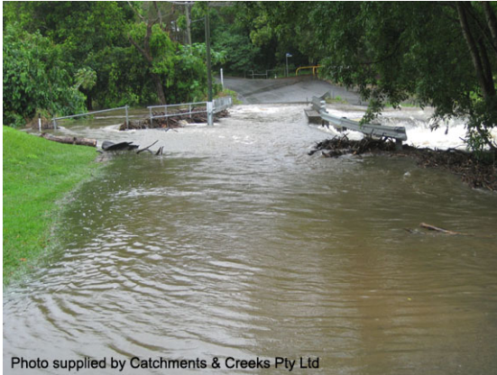
Flooded road crossing
