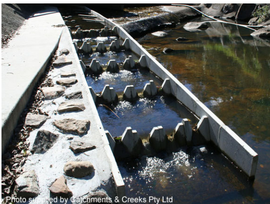
Block-ramp fishway (Walaman)
