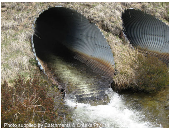
Culvert with drop outlet
