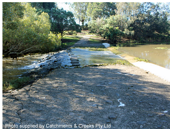
Fish barrier (weir) on main waterway
