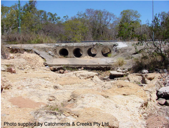
Culvert with elevated apron
