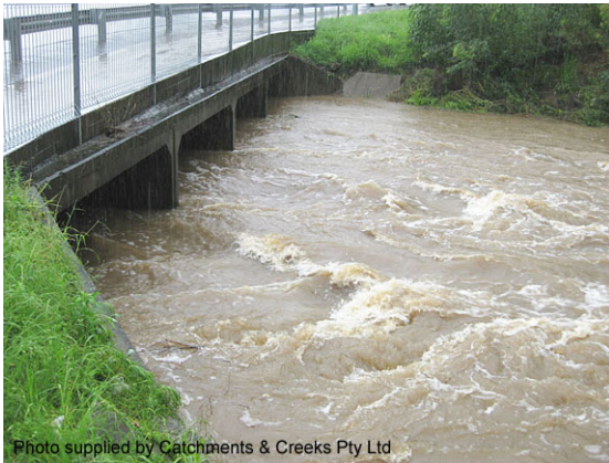
Culvert operation under outlet control
