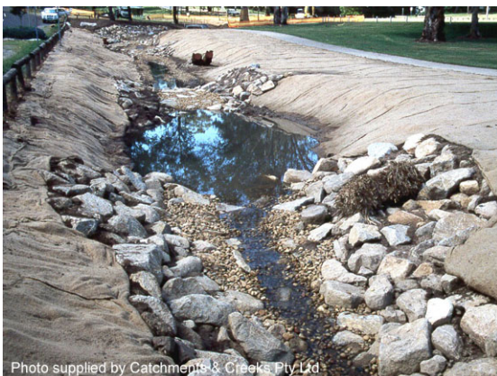
Constructed pool-riffle channel bed
