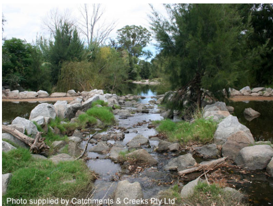
Low-maintenance rock ramp fishway
