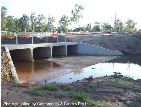
Concrete apron at culver inlet
