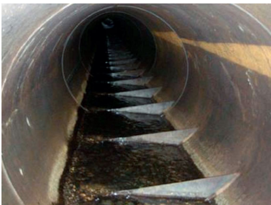
Angled baffles in a pipe culvert
