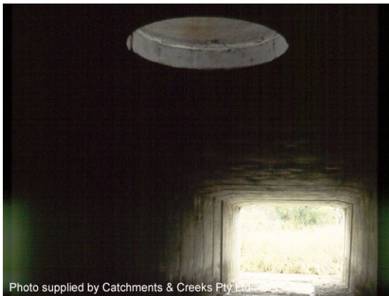
Central skylight in a box culvert
