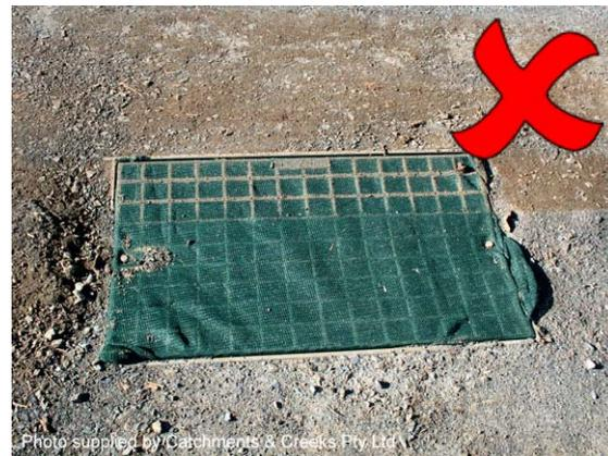
**Photo 2 – Shade cloth should not be used, also note no sediment collection trench formed around the drop inlet**
