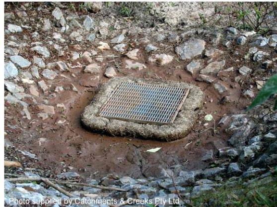
**Photo 2 – Fibre roll supplementary sediment trap around a field (drop) inlet**
