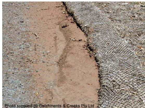
**Photo 6 – Fibre roll damaged (flattened) by traffic, but still functional**
