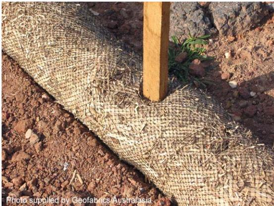
**Photo 1 – Fibre roll staked across a uniform slope**
