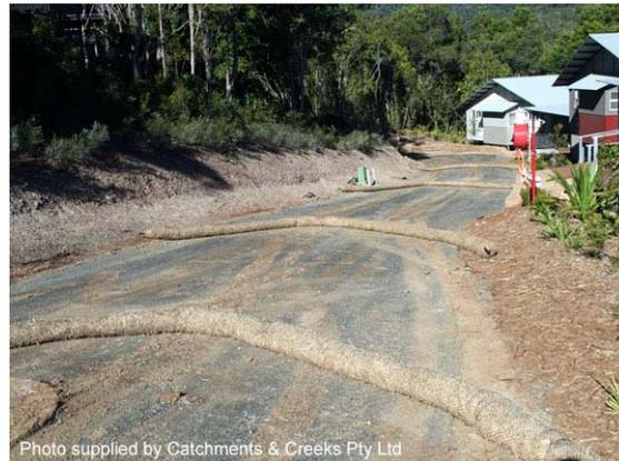
**Photo 4 – Fibre rolls used as an end-of-day flow and sediment control system**
