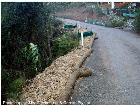
**Photo 5 – Fibre rolls used as a minor sediment trap and flow protection for the adjacent mulched batter**
