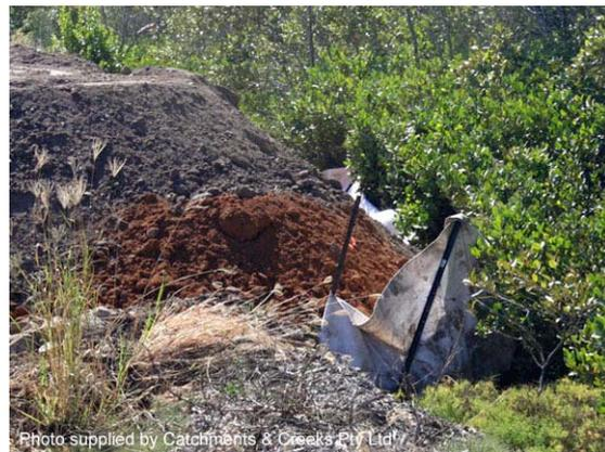
Photo 2 – Filter fence placed down-slope of earth stockpile
