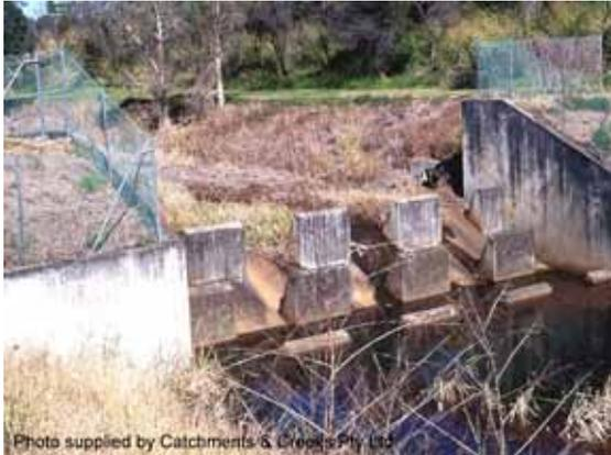
Photo 11 – Baffled spillway
