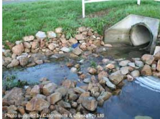
Photo 4 – Rock pad outlet structure
