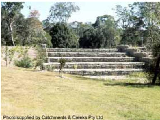
Photo 9 – Gabion lined stepped spillway on a stormwater detention basin
