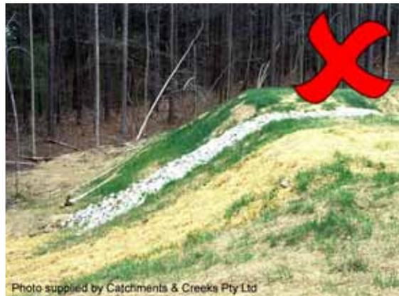
Photo 14 – A suitable energy dissipater must be constructed at the base of the spillway
