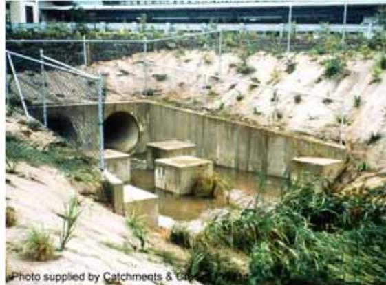
Photo 12 – Impact block energy dissipater
