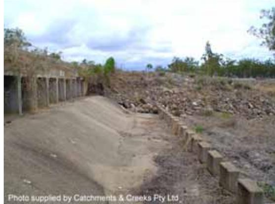
Photo 8 – Note use of impact blocks to stabilise the location of the hydraulic jump
