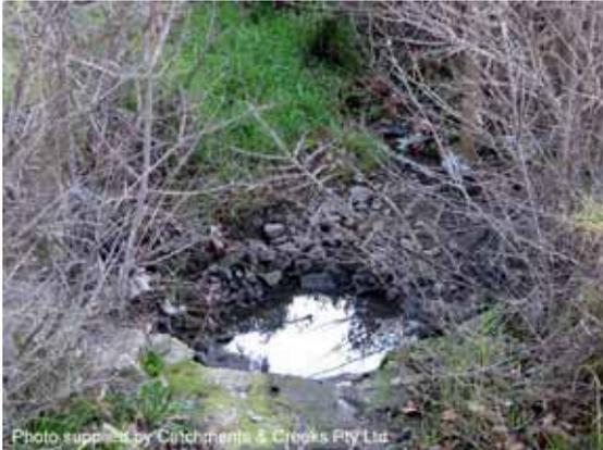
Photo 7 – Rock-lined plunge pool energy dissipater
