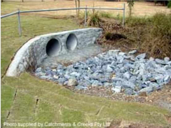
Photo 3 – Rock pad outlet structure
