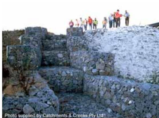
Photo 10 – Stepped chute acting as an outlet structure for a table drain
