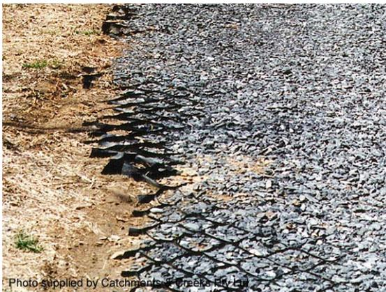
**Photo 1 – Cellular confinement system used to restrict gravel movement on a permanent car park**
