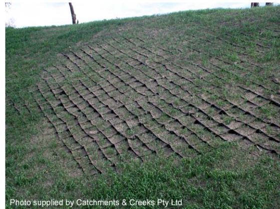
**Photo 2 – Cellular confinement system used to retain soil and assist in the establishment of grass on a steep slope**
