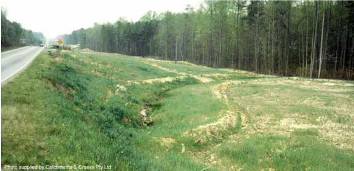
**Photo 7 – Flow diversion banks placed each side of drainage line passing through road construction site**
