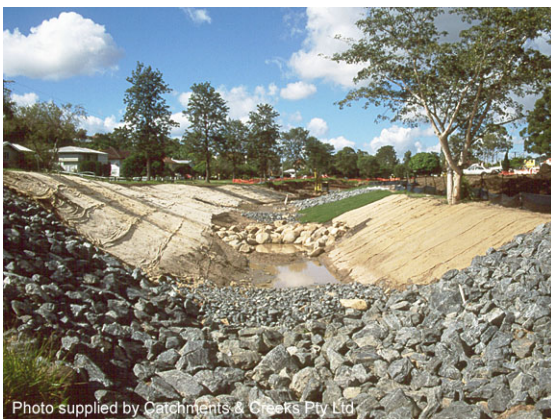
Looking u/s from d/s end of works (2000)
