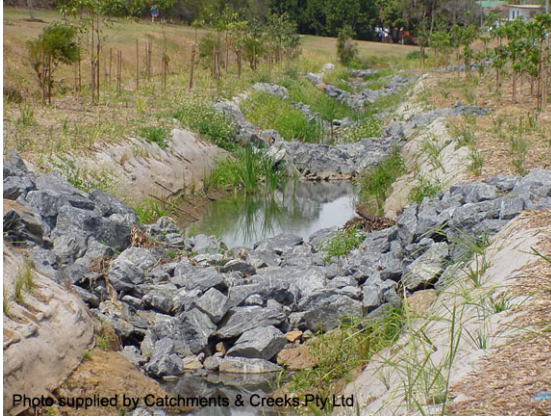
Constructed pool-riffle system (2001)
