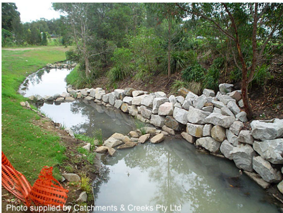
Looking downstream from outlet (2005)
