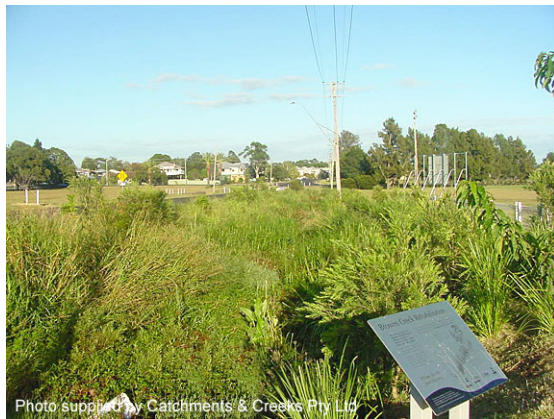
Looking down drainage channel (2005)
