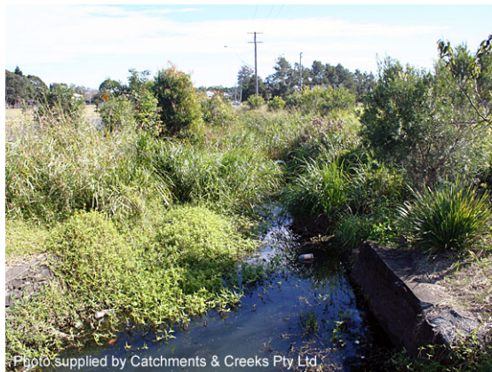
Looking down drainage channel (2007)
