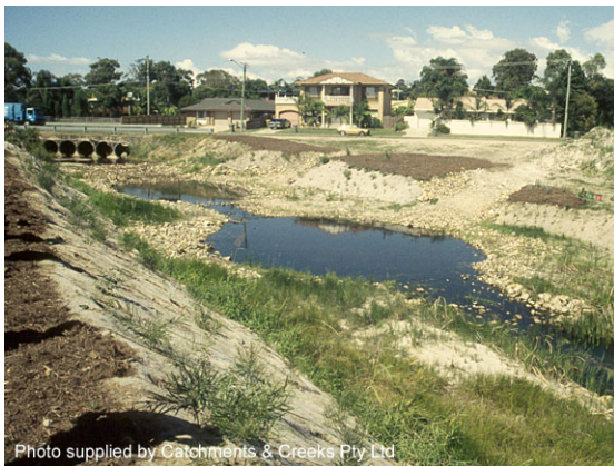
Sediment pond upstream of works (1996)
