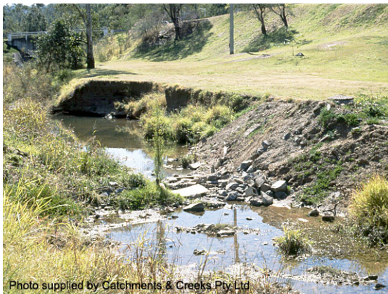
Protection of sewer with rubble (1991)
