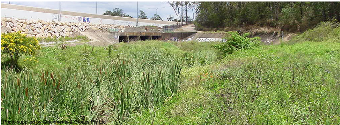
Looking downstream to culvert (2000)
