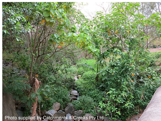
Looking u/s from d/s end of works (2014)
