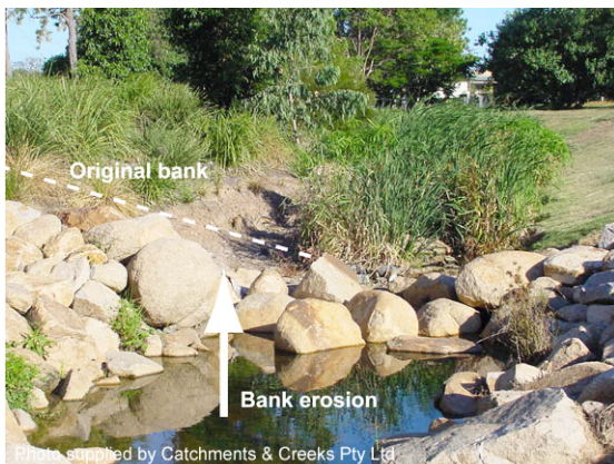
Bank erosion adjacent rock riffle (2002)
