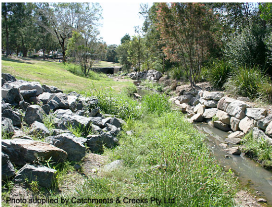
Looking d/s towards end of works (2008)
