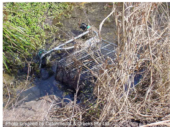
Deposition of rubbish in storm drain
