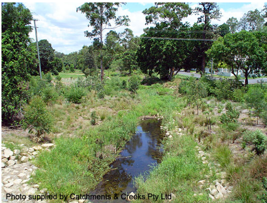
Looking d/s from Moggill Rd (2004)
