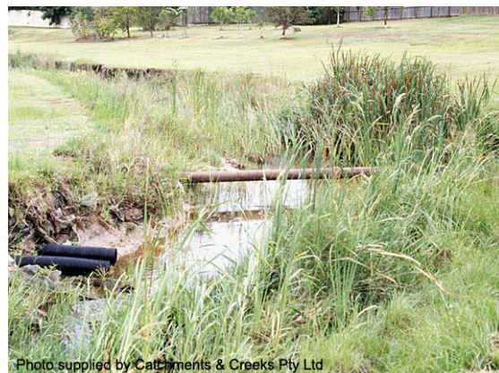
Exposed Ag-pipe & sewer crossing (1997)
