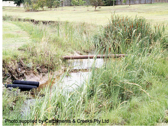
Sewer pipe crossing (1997)
