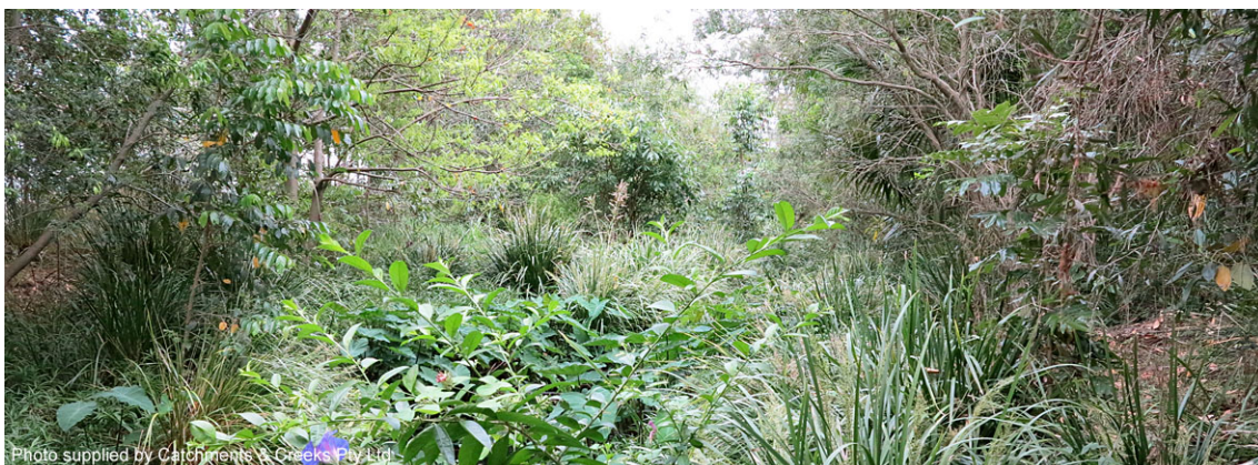
Looking downstream to culvert (2014)
