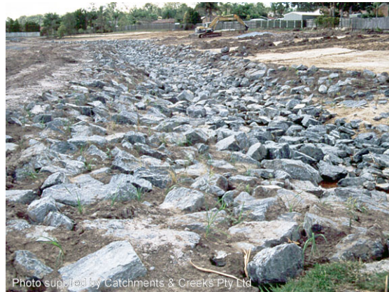
Sewer pipe crossing (1999)
