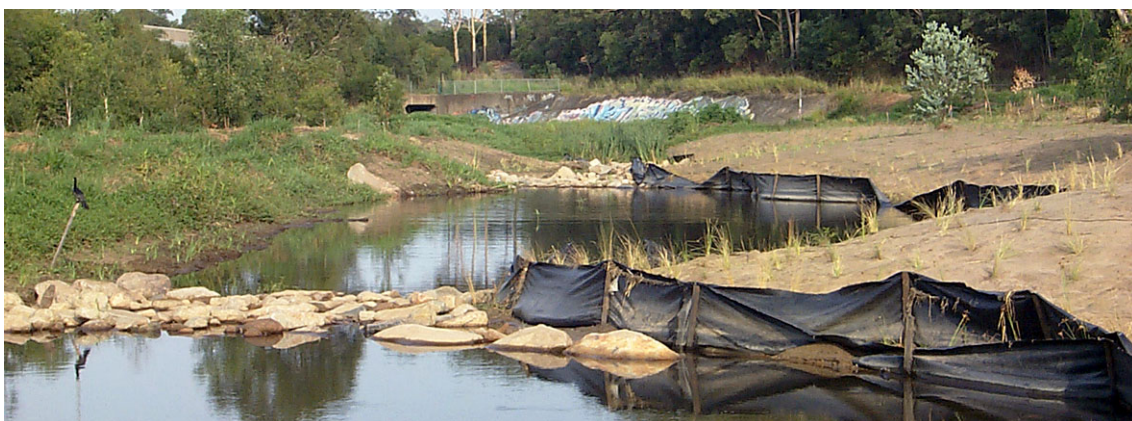
Looking downstream to culvert (2001)
