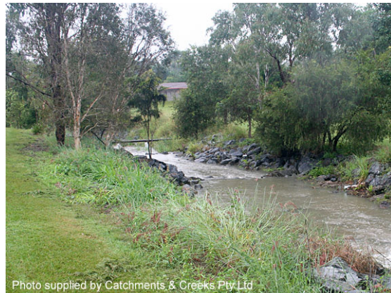
Sewer pipe crossing (2010)
