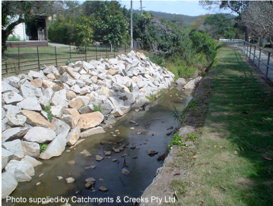
Upstream end of works (2005)
