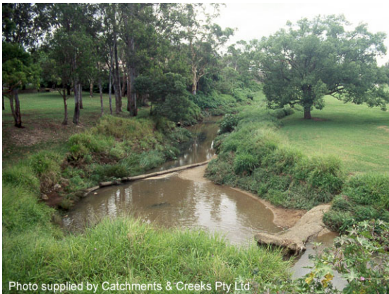
Looking downstream from bridge (1998)
