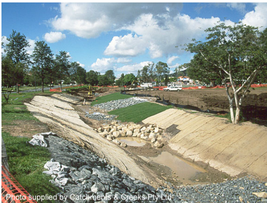
Looking u/s, d/s from junction (2000)
