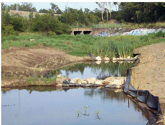
Looking downstream to culvert (2001)
