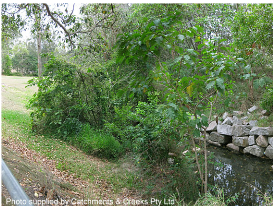
Looking downstream from outlet (2014)
