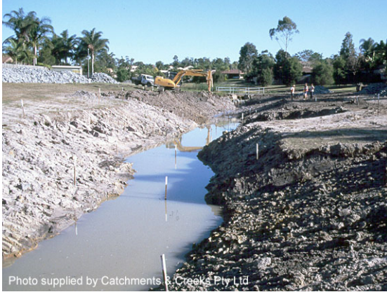
Looking u/s, construction phase (1999)
