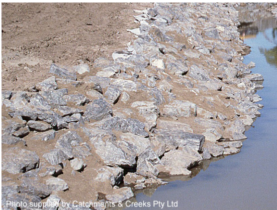
Soil-filled voids ready for planting (1999)
