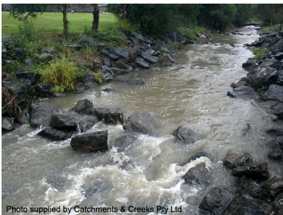
Pool-riffle system (2010)
