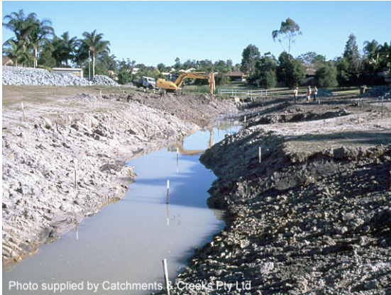
Major creek rehabilitation project
