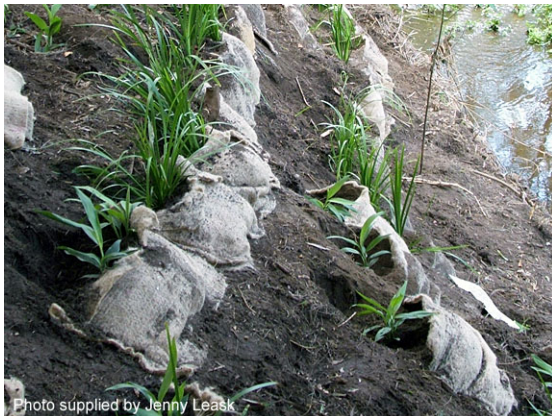
Jute bagging planting technique (2005)
