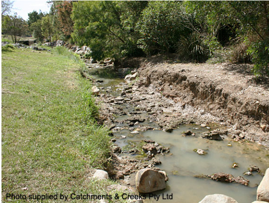
Looking d/s towards end of works (2008)
