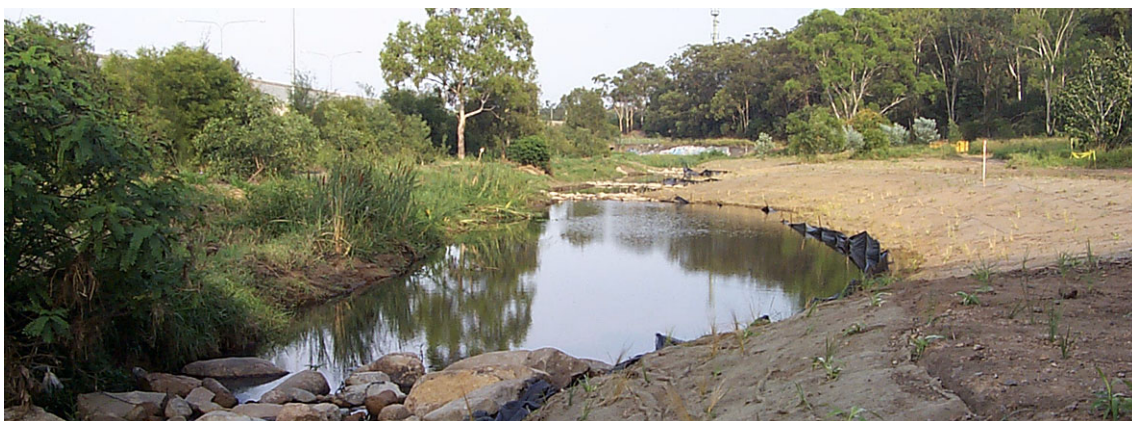
Looking downstream to culvert (2001)
