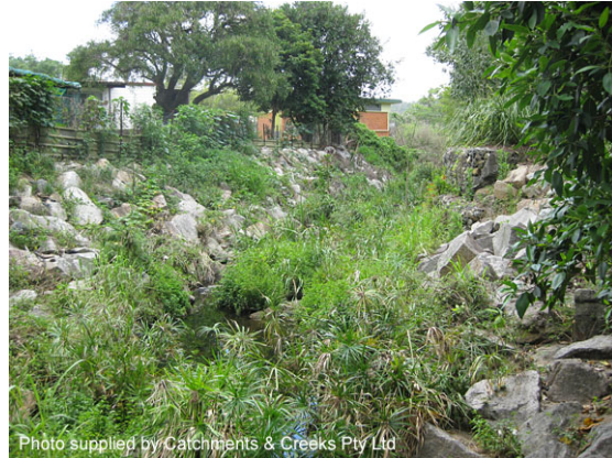
Upstream end of works (2012)
