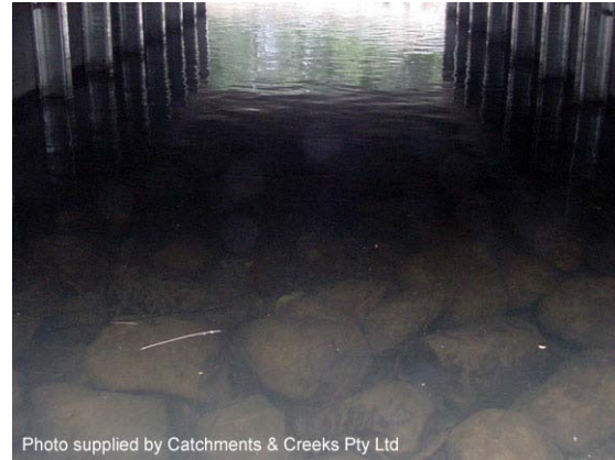
Photo 2 – Added culvert bed roughness
