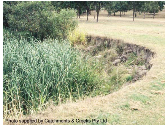
Photo 2 – Bank scour around the outside of a channel bend (Qld)
