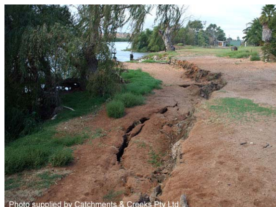
Photo 3 – Bank slumping (SA)
