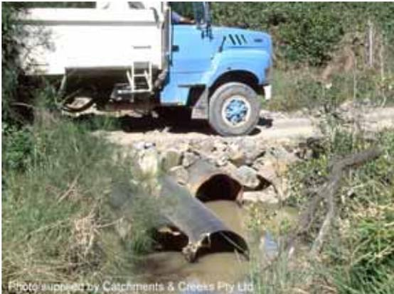
**Photo 1 – Temporary culvert formed from recycled steel pipes**
