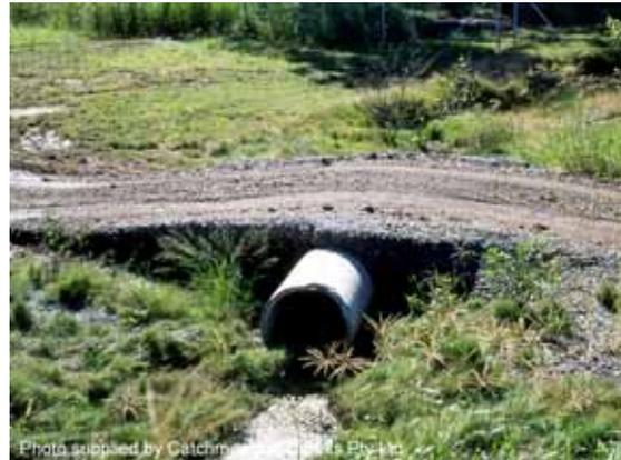
**Photo 2 – Temporary crossing of minor drainage channel**
