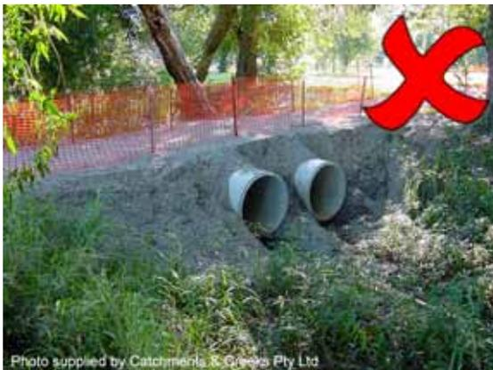
**Photo 3 – Using only fine aggregate to form the fill embankment can result in severe wash-outs if overtopped**
