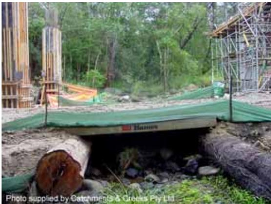
**Photo 1 – Temporary bridge crossings formed with 'bridging slab'**
