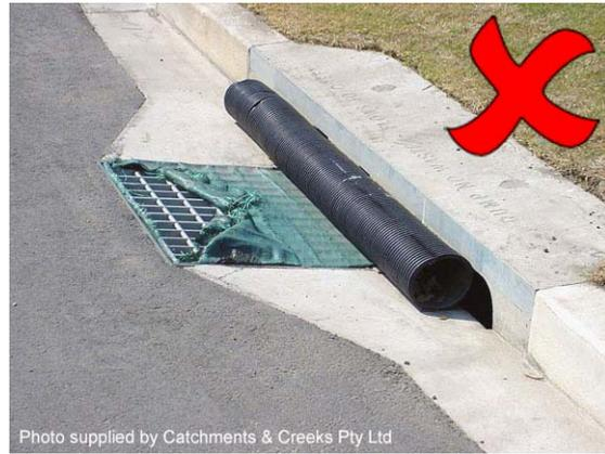
**Photo 8 – The sediment barrier should not block the stormwater inlet**
