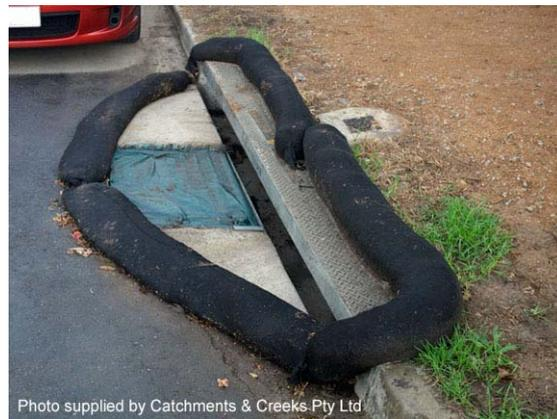
**Photo 2 – Use of filter socks to form a sediment trap at a sag inlet**
