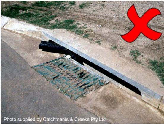
**Photo 7 – ‘Spacers’ should be used to separate the sediment barrier from the kerb inlet and prevent the barrier from being washed into the inlet**
