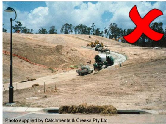
**Photo 10 – Straw bales should not be placed on solid surfaces**
