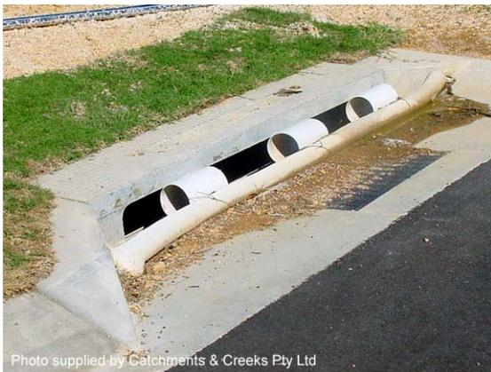
**Photo 1 – Protected 'sag' inlet (note the use of 'spacers' to keep the inlet open)**
