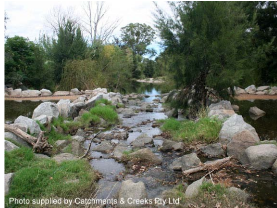
Photo 2 – Constructed fishway ramp
