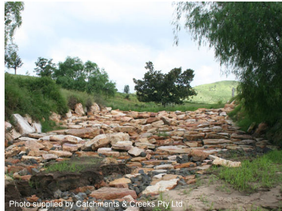
Photo 2 – Rock-lined gully chute
