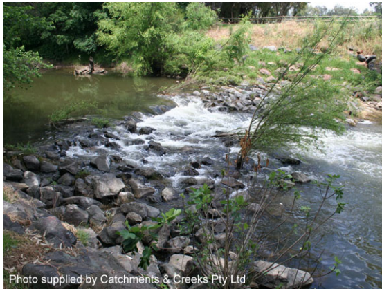
Photo 1 – Rock-lined waterway chute
