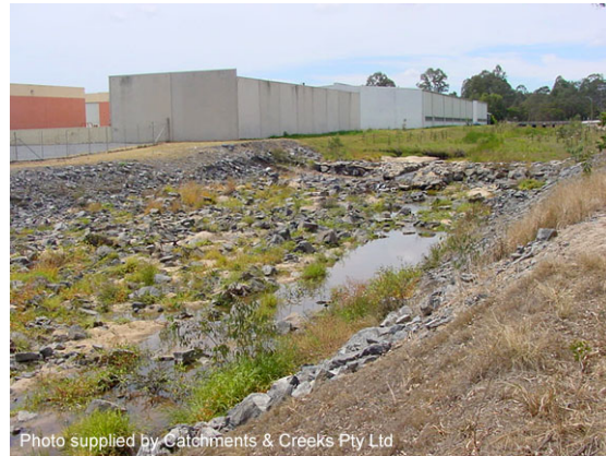
Photo 2 – Rock-lined grade control (drop) structure
