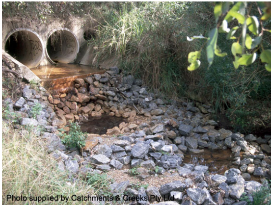
Photo 1 – Plunge pool energy dissipater outlet structure
