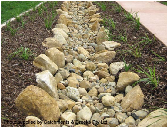
Photo 1 – Rock-lined drainage channel
