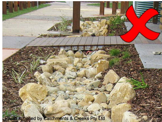
Photo 6 – During construction, the drain should be excavated sufficiently to allow placement of the rock such that the finished drain has the required flow area
