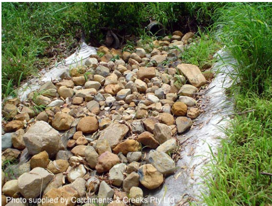
Photo 5 – Rounded rock can be significantly less stable than angular, fractured rock, especially when placed on steep slopes
