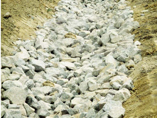
Photo 3 – Placement of the rock on the soil can result in erosion problems if significant lateral inflows occur
