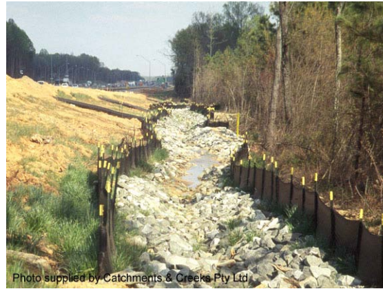
Photo 2 – Rock-lined catch drain (during construction phase)
