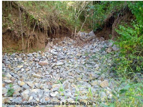
Photo 2 – Rock-lined drainage chute used in the stabilisation of a gully
