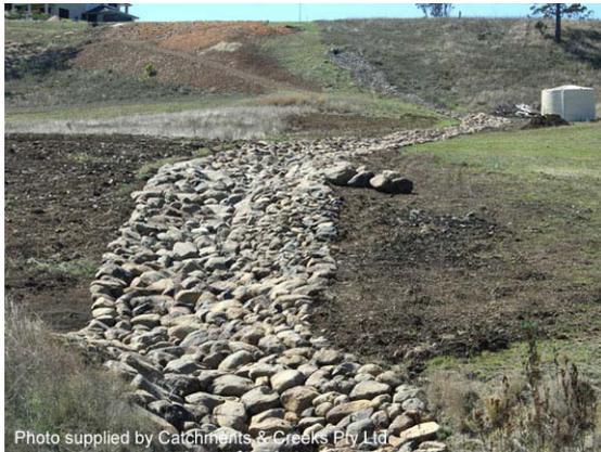
Photo 1 – Rock-lined drainage chute
