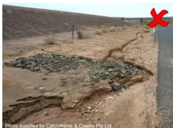
**Photo 10 – Typical erosion problem when placed in dispersive soil**
