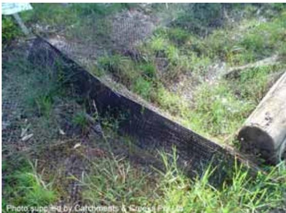
**Photo 5 – Triangular ditch checks**
