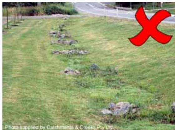
**Photo 8 – Retained rock check dams can interfere with ongoing mowing**
