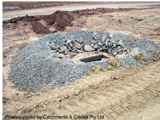
**Photo 2 – Rock and aggregate drop inlet protection**
