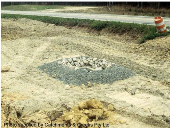
**Photo 1 – Rock and aggregate drop inlet protection located with dual carriageway**
