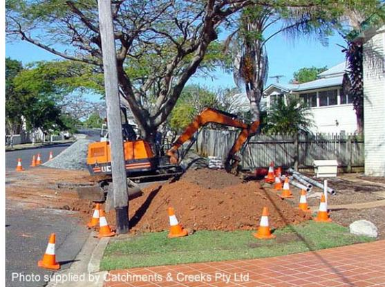
**Photo 2 – Installation of new sewer connection**
