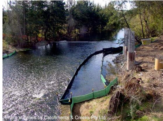
**Photo 2 – Sediment fence isolation barrier**
