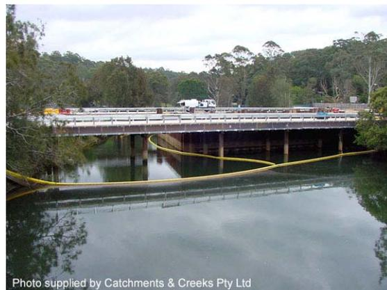
**Photo 4 – Sheet piling used to form a dry work area with the floating silt curtains used as a sediment containment system**
