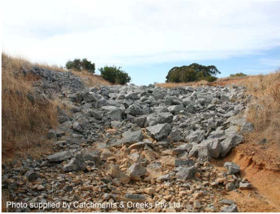
Photo 3 – Rock chute showing flat crest (note; the rock has not been extended sufficiently up the sides of the chute, SA)
