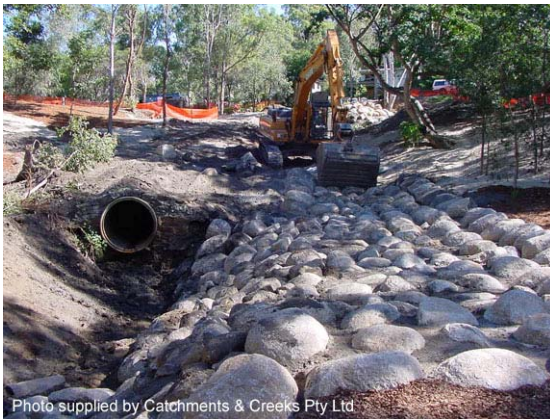
Photo 5 – Construction of rock chute with voids filled with soil (Qld)
