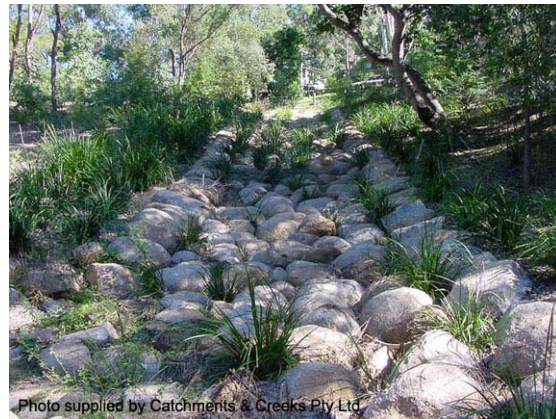
Photo 6 – Same chute (left) with plants established within voids (Qld)
