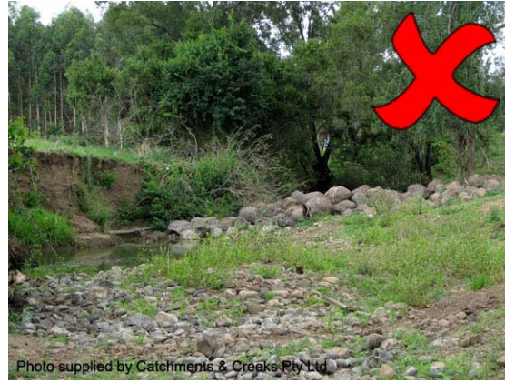
Photo 4 – Rock chute with the crest sloping to the left resulting in bank erosion (visible on left, Qld)
