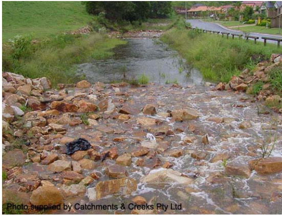
Photo 1 – A series of short rock chutes constructed within a stormwater drain (Qld)
