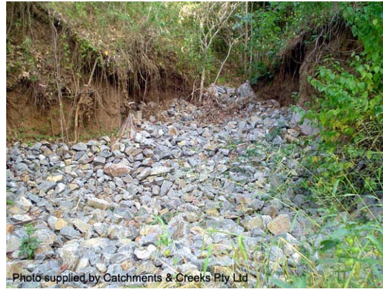
Photo 2 – Rock chute formed at the head of an urban gully (Qld)
