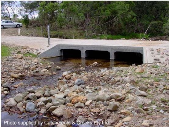
**Photo 1 – Recessed box culvert**
