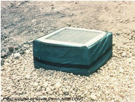
**Photo 1 – Fabric drop inlet protection incorporating a timber support frame**
