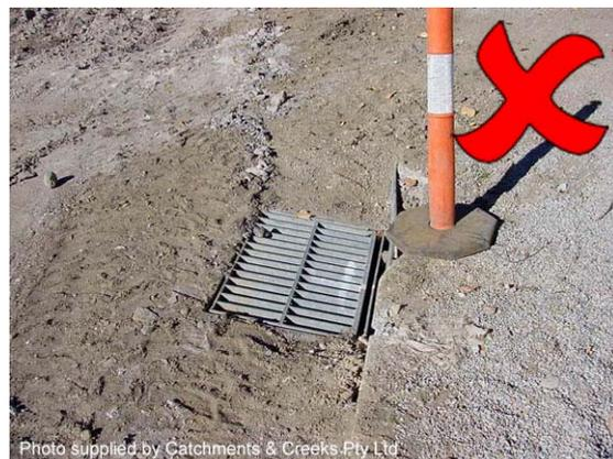
**Photo 4 – Stormwater inlet with no sediment protection**
