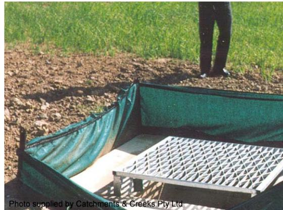
**Photo 2 – Fabric drop inlet protection (note, support stakes are too far apart)**
