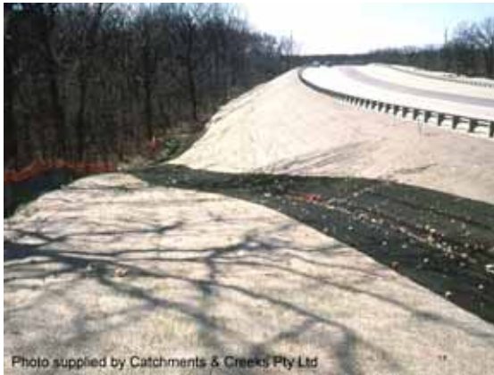
Photo 1 – Application of erosion control blankets and mats
