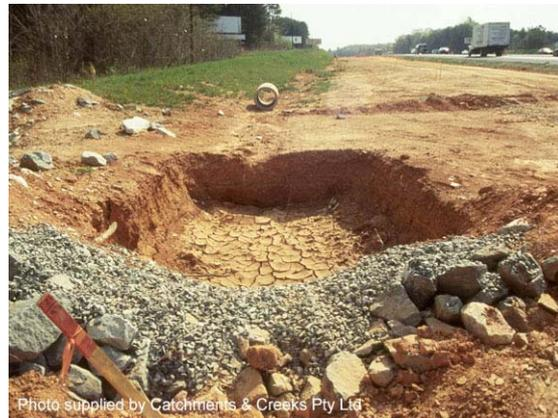
Photo 2 – Temporary excavated sediment trap up-slope of a *Rock Check Dam*
