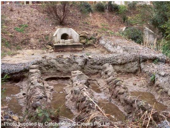
Photo 1 – Permanent excavated sediment trap on a stormwater outlet
