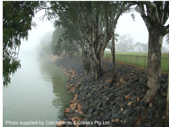
Photo 2 – Rock stabilisation of a river bank
