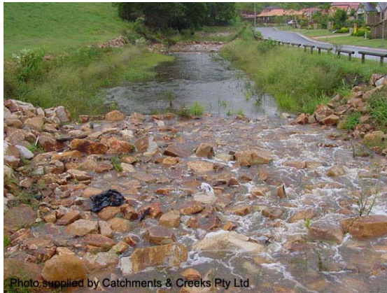
Photo 1 – Rock-lined grade control structure
