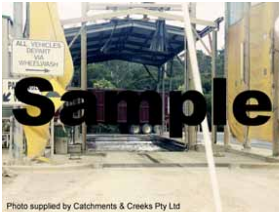
Photo 1 – Permanent, automatic wash bay located on site
