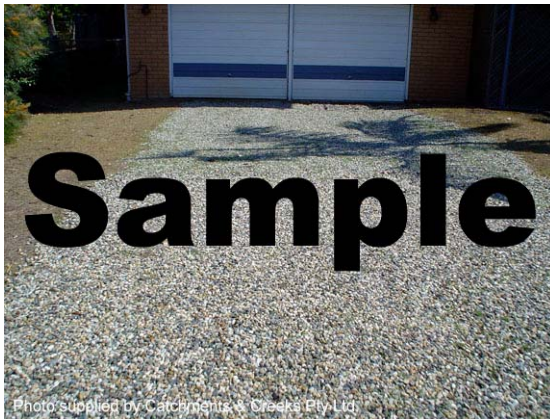
Photo 1 – Stage 1: placement of aggregate
