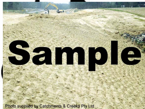
Photo 2 – Corrugated (roughened) surface
