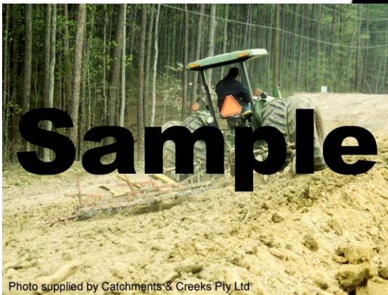
Photo 7 – Contour ploughing
