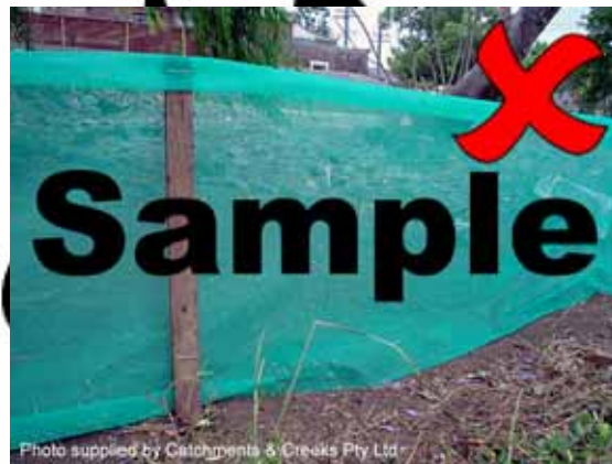
Photo 4 – Composite sediment fence (not preferred)
