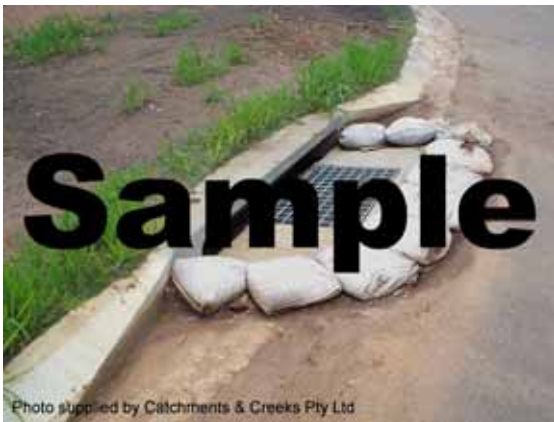
Photo 5 – sandbag curb inlet protection
